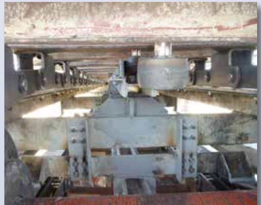
THIELE roller installed as a central guide unit on a threaded bolt.
